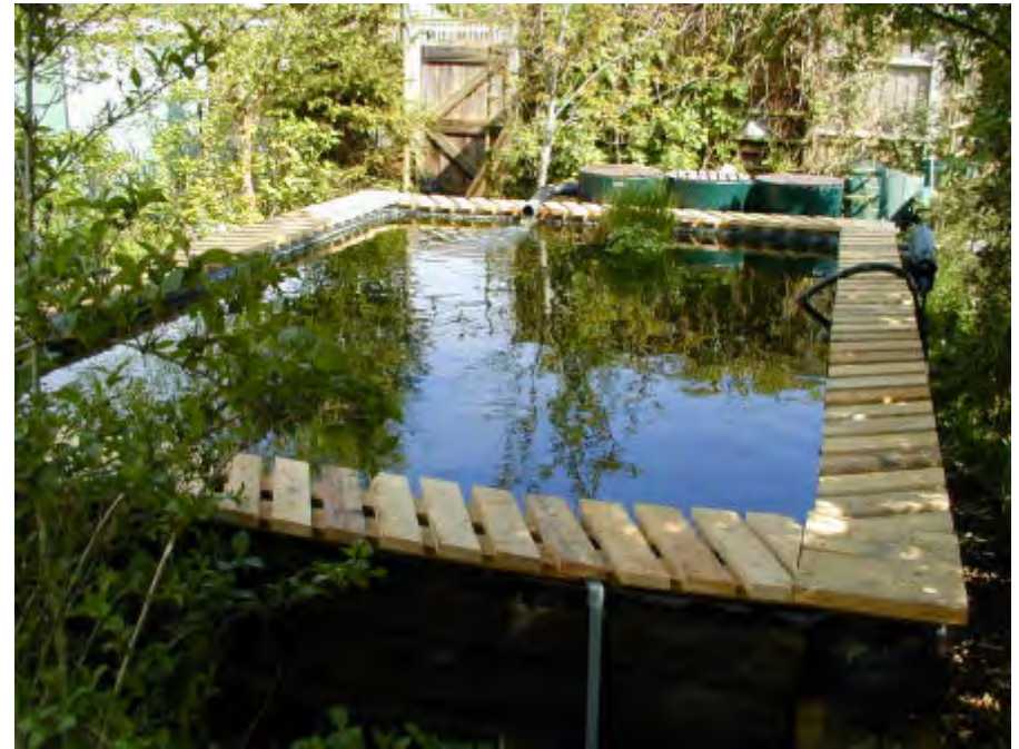
The pond in late April 2000, after a mild winter, and with the coping on the walls just completed. The slat-work is made from untreated, air-dried oak, 3x1", set 1" apart and at a 30° angle; the slats are screwed onto rails of the same timber.
