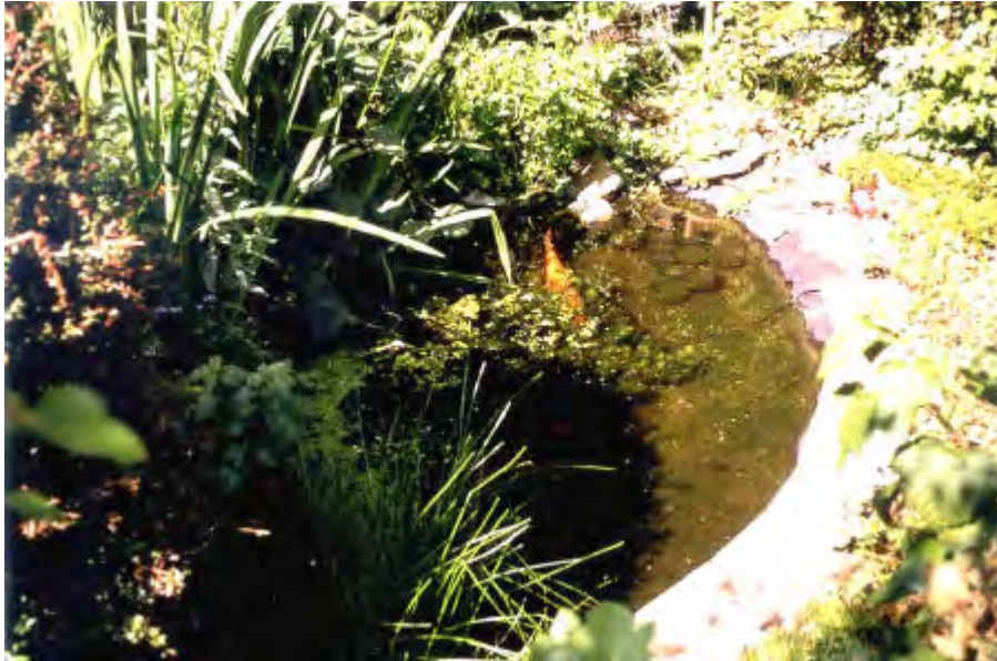
The old pond, before work started: overgrown and too small for large koi - although a good wildlife habitat.
