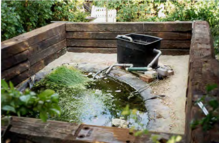
Completed sleeper construction showing old pond and filter still in place
