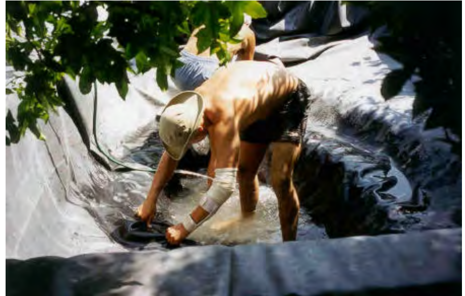
Fitting the liner: as the water is added it is essential to ensure all the folds are neat and tidy; this means one or two people in the water! [Keith (foreground) and Ken]
